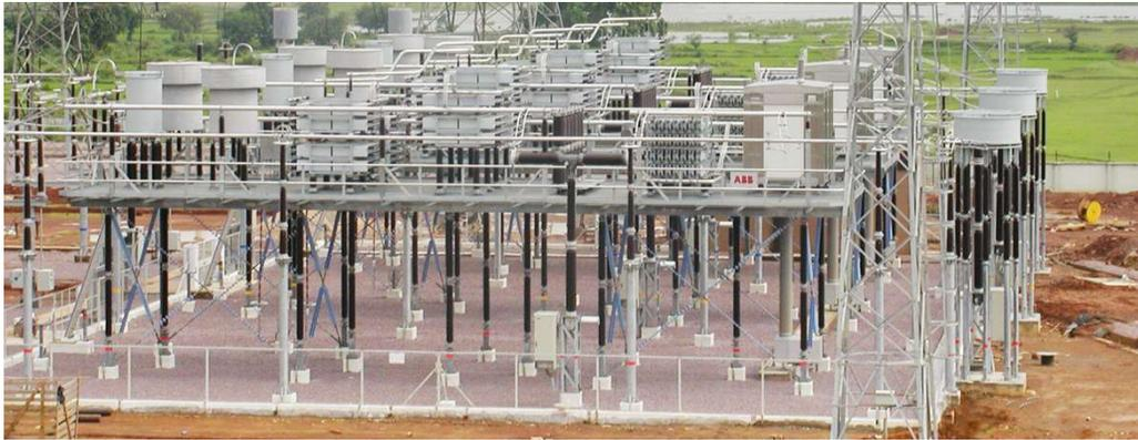
Figure 8.2: TCSC for stable transmission of surplus power from Eastern to Western India from [2].
