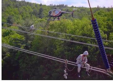
(e) Inspection of high-power lines by linemen in Faraday suits [World Channel, 2016]
