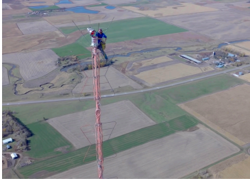
(d) Replacement of the light bulb at the 457 meter TV tower [Prairie Aerial, 2014]
